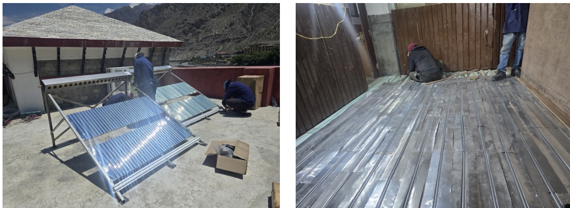
Fig. 3: Installation of solar thermal collectors (left) and of the floor heating system (right). (Source: Dibya Acharya)
