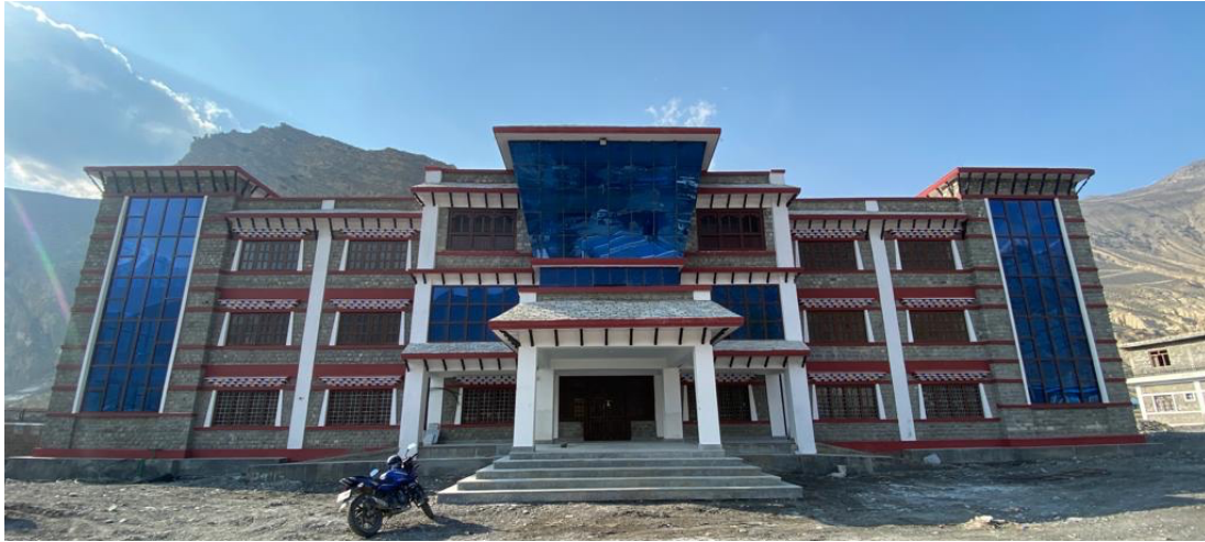
Fig. 1: Frontview of the Gharapjong municipality office building in Jomsom, Mustang, Nepal. (Source: Michael Strobel)
