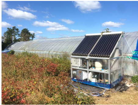
Fig.2 : Picture of developed hybrid heat pump system in the empirical site and Dimension of greenhouse
