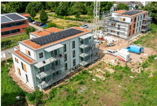
Fig. 4: Completed MFH with PVT collectors on the roof; both buildings (left) and PVT modules/field from the roof (right)
