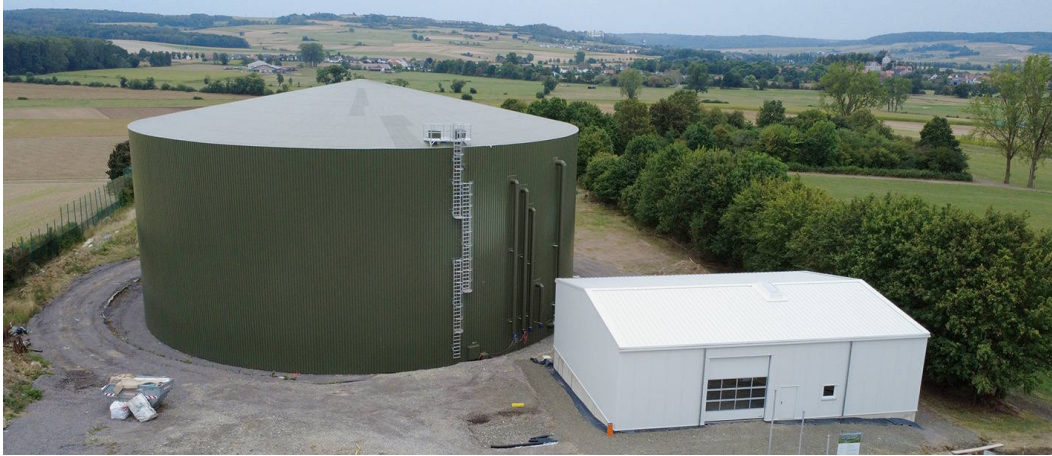
Fig. 12: Completed seasonal storage tank with energy central.
