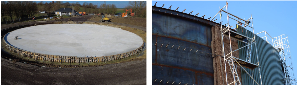
Fig. 11: Foundation (left) and insulation (right) during construction of the seasonal storage tank.
