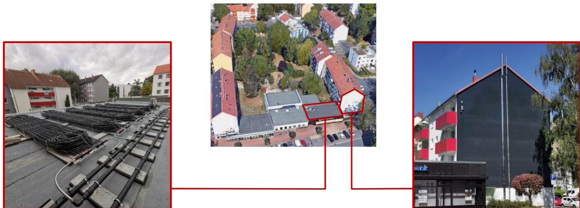
Fig. 2: Demonstration building with thermally active metal façade. General view of the building complex under renovation (center), installed solar air absorber field (left) and active metal façade (right).
