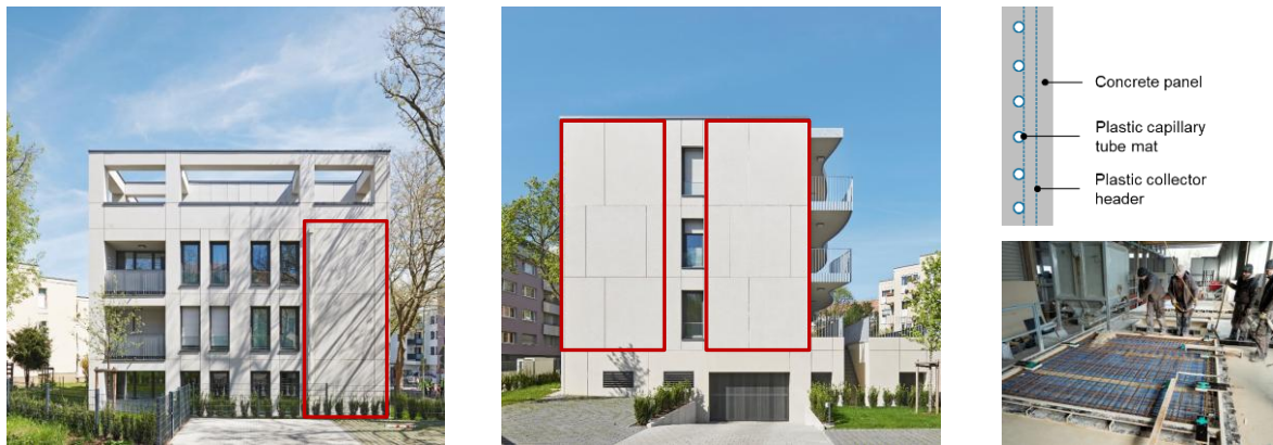
Fig. 1: Demonstration building with thermally active concrete façade. View of the west (left) and east (center) façades as well as design sketch and manufacturing process (right)
