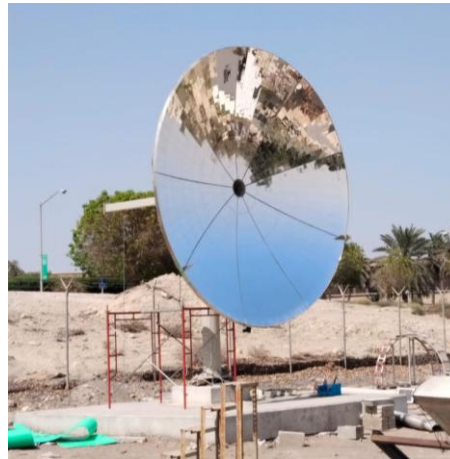
Fig. 2 The dish after installation on site
