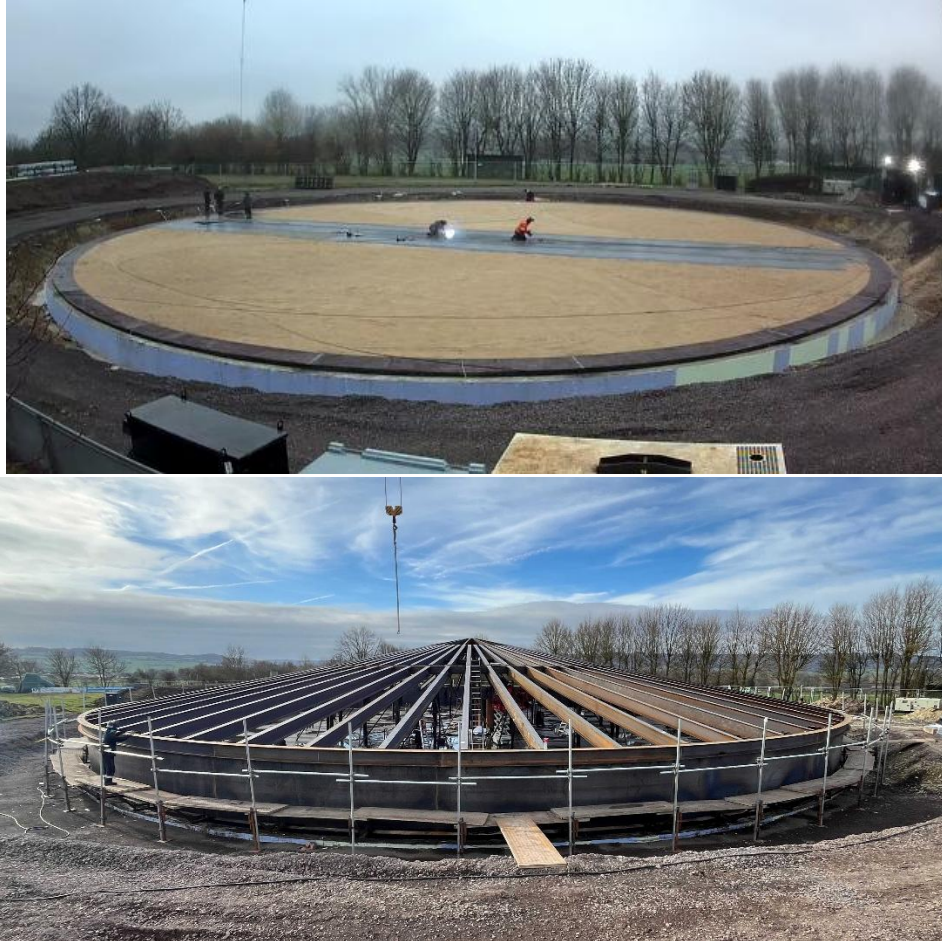
Fig. 3: Current (March 2026) status of construction – storage base plate (top) and top cover (bottom) construction
