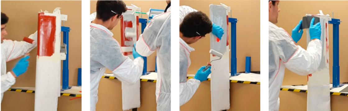
**Figure 6.** Leading Edge Protection Service application with different techniques, from left to right: application of the primer layer, the putty/filler/LEP material, thickness needs to be monitored closely, the surface is screened down to ensure a flat, smooth surface following the blade contour
