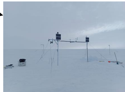
Installed from January 10 to 15, 2026
