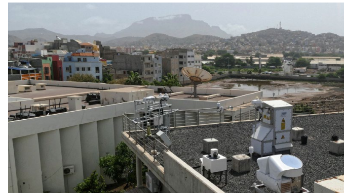
Aerosol, cloud and radiation station on the roof of the Ocean Science Center Mindelo, Cabo Verde (Rico Hengst, TROPOS)
