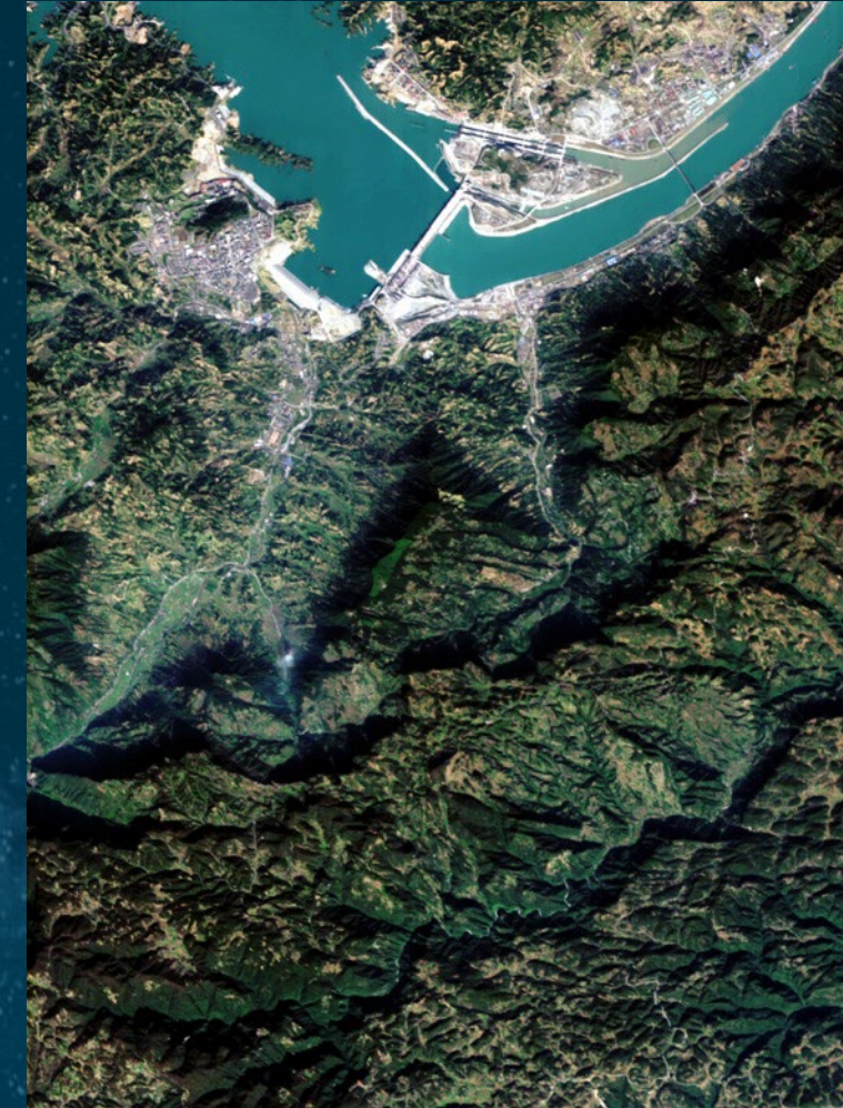
Three gorges dam (China)
