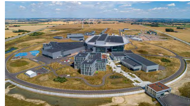
ESS, Lund, Sweden, Under construction
