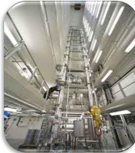
Tiller Pilot Plant
