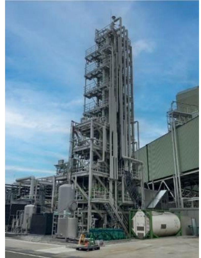
Himeji CO 2 Capture Pilot Plant
