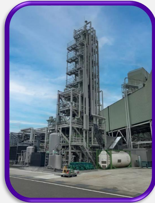
Himeji CO 2 Capture Pilot Plant, 5 tonnes/day, (Mitsubishi, 2025)
