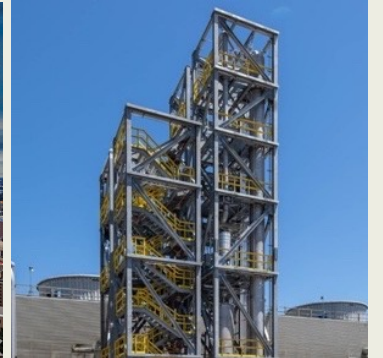
ION Pilot Plant in Pittsburg, CA
