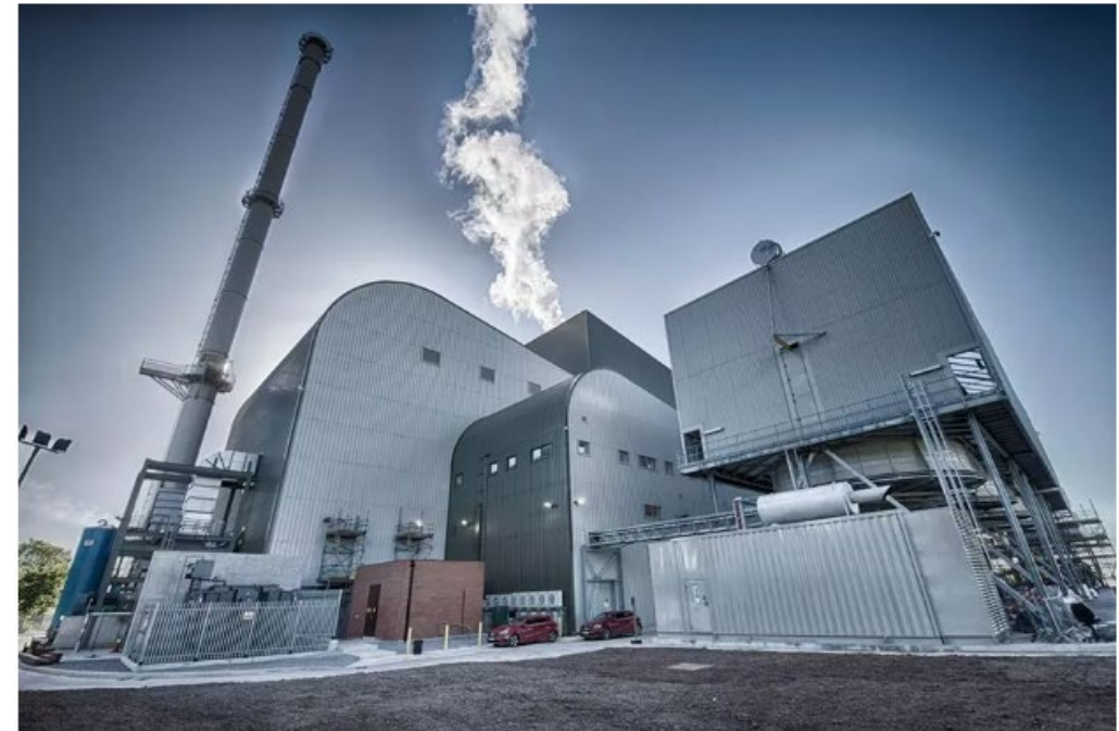
Ince Bio Power (Photo courtesy of Evero Energy Group)
