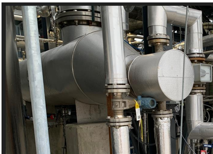
Figure 4: Kettle reboiler at TERC (L) and once-through thermosyphon reboiler at Haifeng pilot (R) – it will be discussed how the type of reboiler used in pilot testing is a critical factor that is often overlooked
