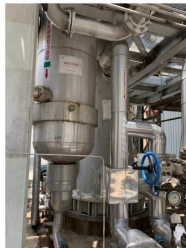
Figure 4: Kettle reboiler at TERC (L) and once-through thermosyphon reboiler at Haifeng pilot (R) – it will be discussed how the type of reboiler used in pilot testing is a critical factor that is often overlooked
