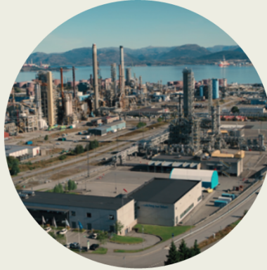
200 TPD CO 2 Project Slingshot
