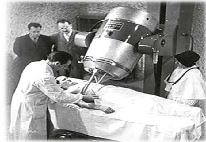
First Cobalt-60 beam machine, 1950-th
