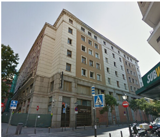
Before office building
