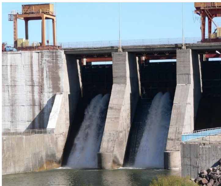
FIGURE 5. Spillway dam on the Astana reservoir.
