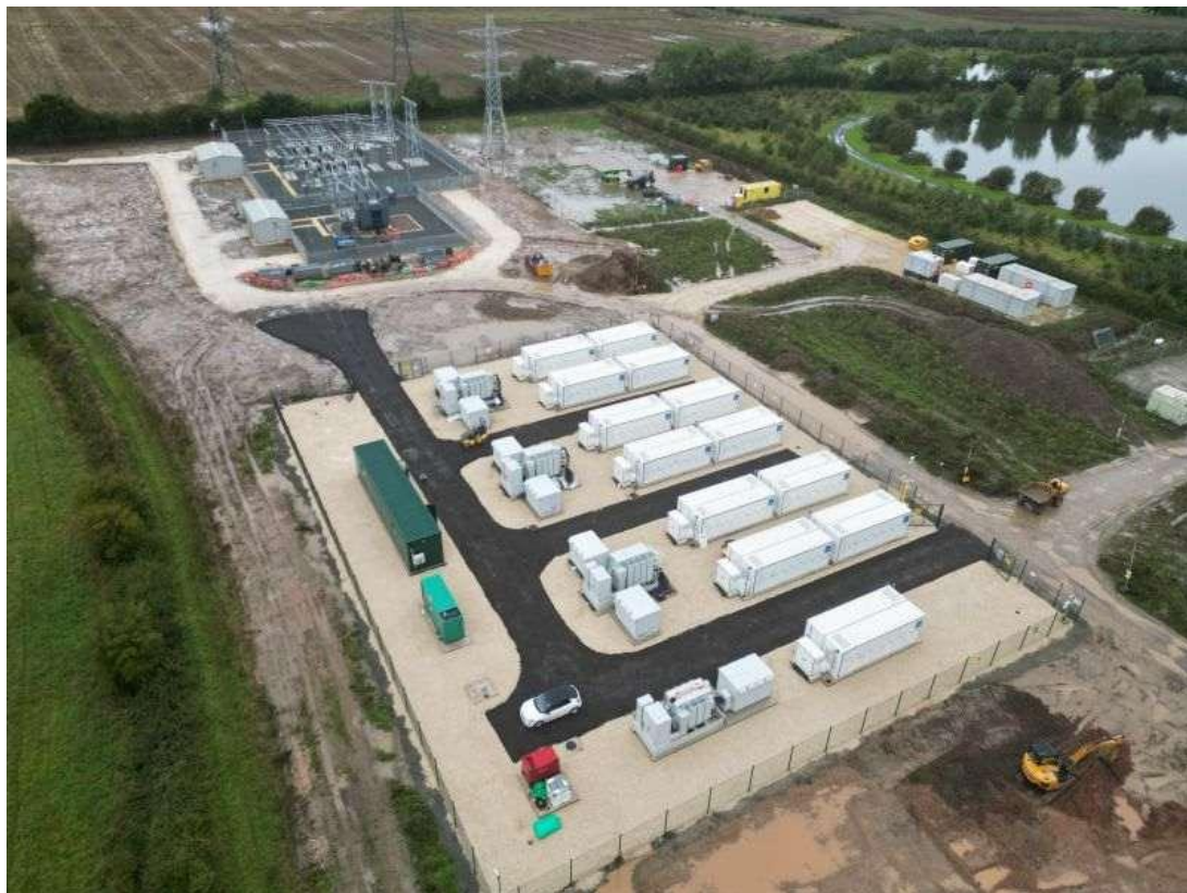
Figure 2: Example of 25MW/50MWh Battery Energy Storage System in the UK (Lightsource bp, 2024)
