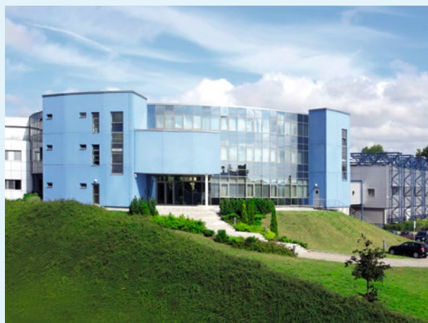
Miltenyi Biotec B.V. & Co. KG, GMP-compliant manufacturing plant, Teterow, Germany
