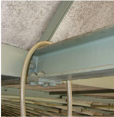
Steel sling at joint.
