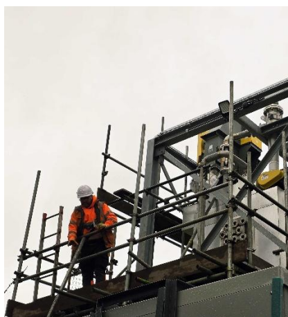
Figure 1 Early-stage installation of the direct air capture pilot plant at the Net Zero Industry Innovation Centre, Teesside.
