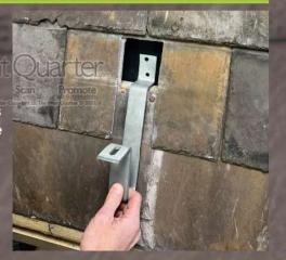
9 Use shims / packings to create clearance between the bracket and the roofing material.
