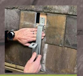
10 Cut down SpeedFlash® to required size (determined by the size of the slate).
