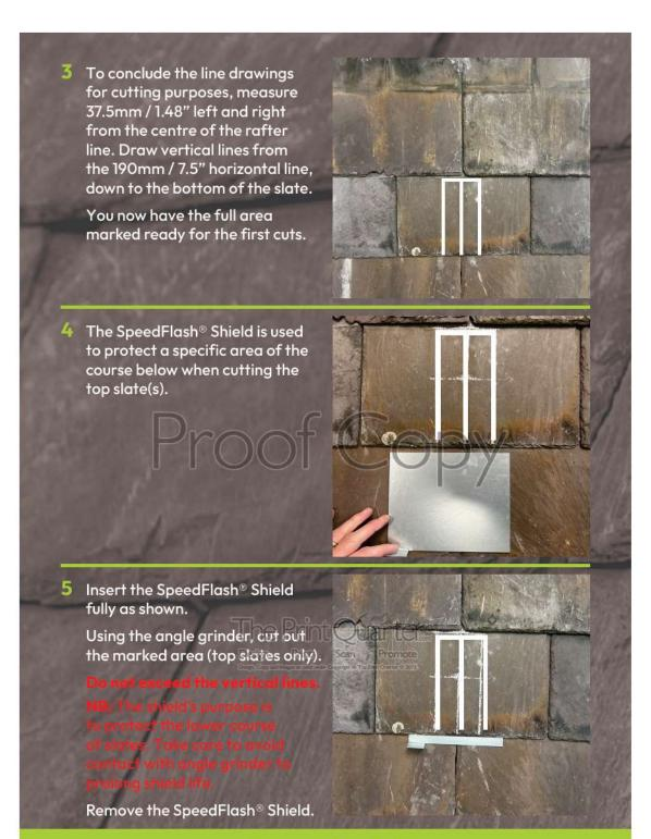
Now you have cut the top slate(s), you need to cut the lower course to create the working area (the area in which the bracket will be fixed).
