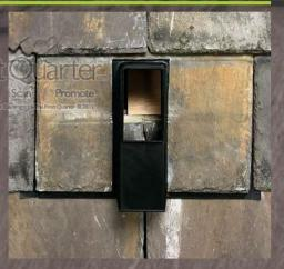
12 To hold the SpeedFlash® in place, use the metal spring support. Insert support via the bottom opening, hooking the support onto the cut under slate.
