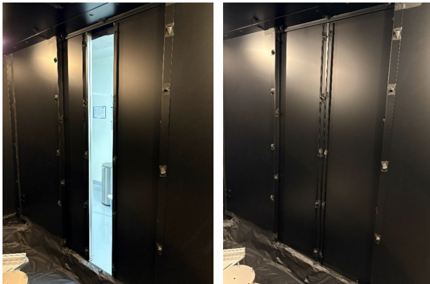
Figure 3-4: View of door (from inside) – open and close
