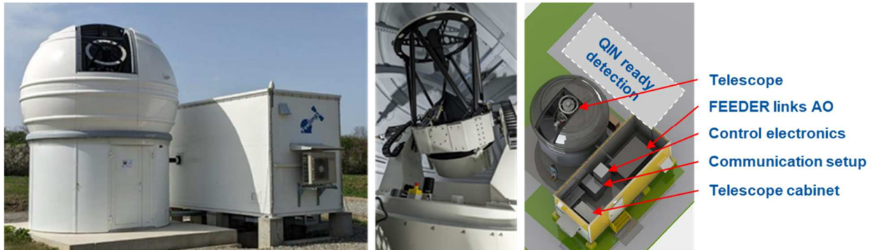
Figure 1 - FEELINGS ground station in Fauga. Dotted line points at available room for an additional Coudé room to host cryogenic detection.
