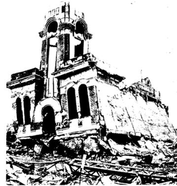
17 psi vs Steel + Reinforced concrete building.
