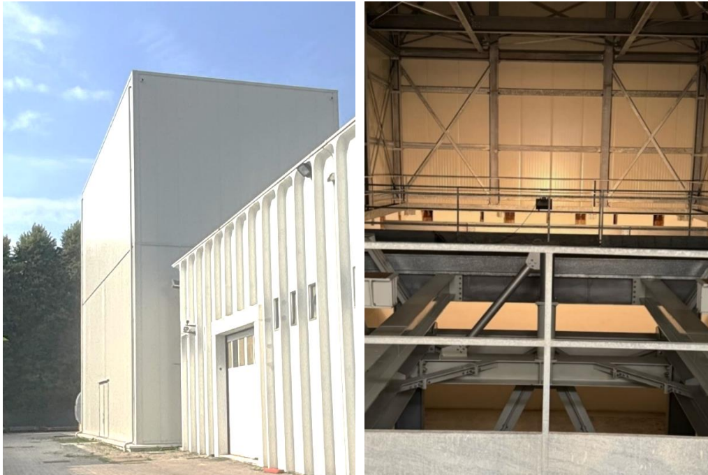
Figure 1. NewATHENA building Exterior (right) and the status of the Interior (left) at Media Lario
