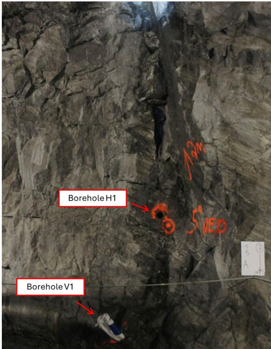
Fig. 3. Photograph of the rock mass with A4 paper for scale and borehole H1 marked with spray paint. Borehole V1 is jammed and stuffed with material visible lower down in the photograph.
