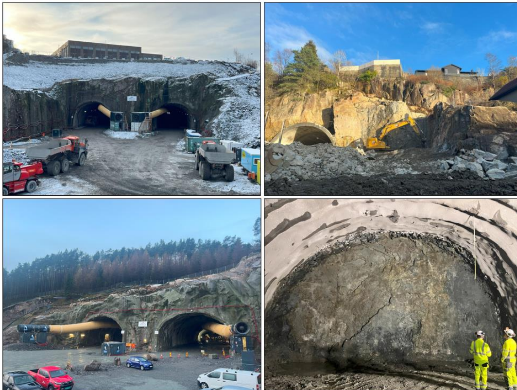
Fig. 2 Straume tunnel East Portal (upper left); The excavation of Kiple GS tunnel West Portal next to the existing Kiple tunnel along Rv.555 (upper right); Drotningstvik tunnel East Portal (lower left); Tunnel face during the excavation of the Kipledalen section (lower right).
