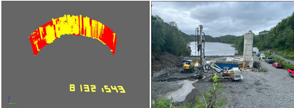
Fig. 8 MWD rock strength data at chainage 8+132 in the North tube (left) and jet-grouting from the surface before the North tube excavation (right).
