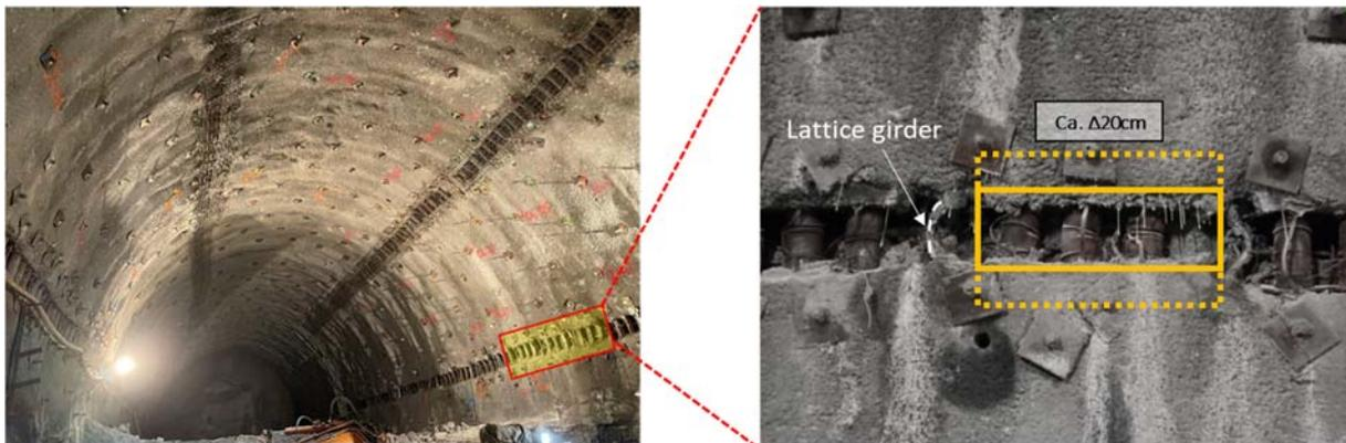
Fig. 5 Tunnel support with 4 rows yielding elements, typ LSC (left) and in detail (right), a approx. 50% compression of the yielding element.
