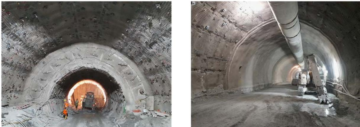
Fig. 7 Tunnel excavation with 10 rows yielding elements and an advanced pilot tunnel (left) and the transition from a ductile support system to a rigid support system with a second shotcrete lining (right)
