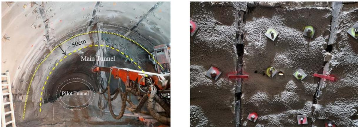
Fig. 10 Reconstruction main tunnel after a displacement  $> 50$  cm and a damaged shotcrete lining (left), HS-EPS yielding elements in the pilot tunnel with a compression  $> 50\%$  (right)
