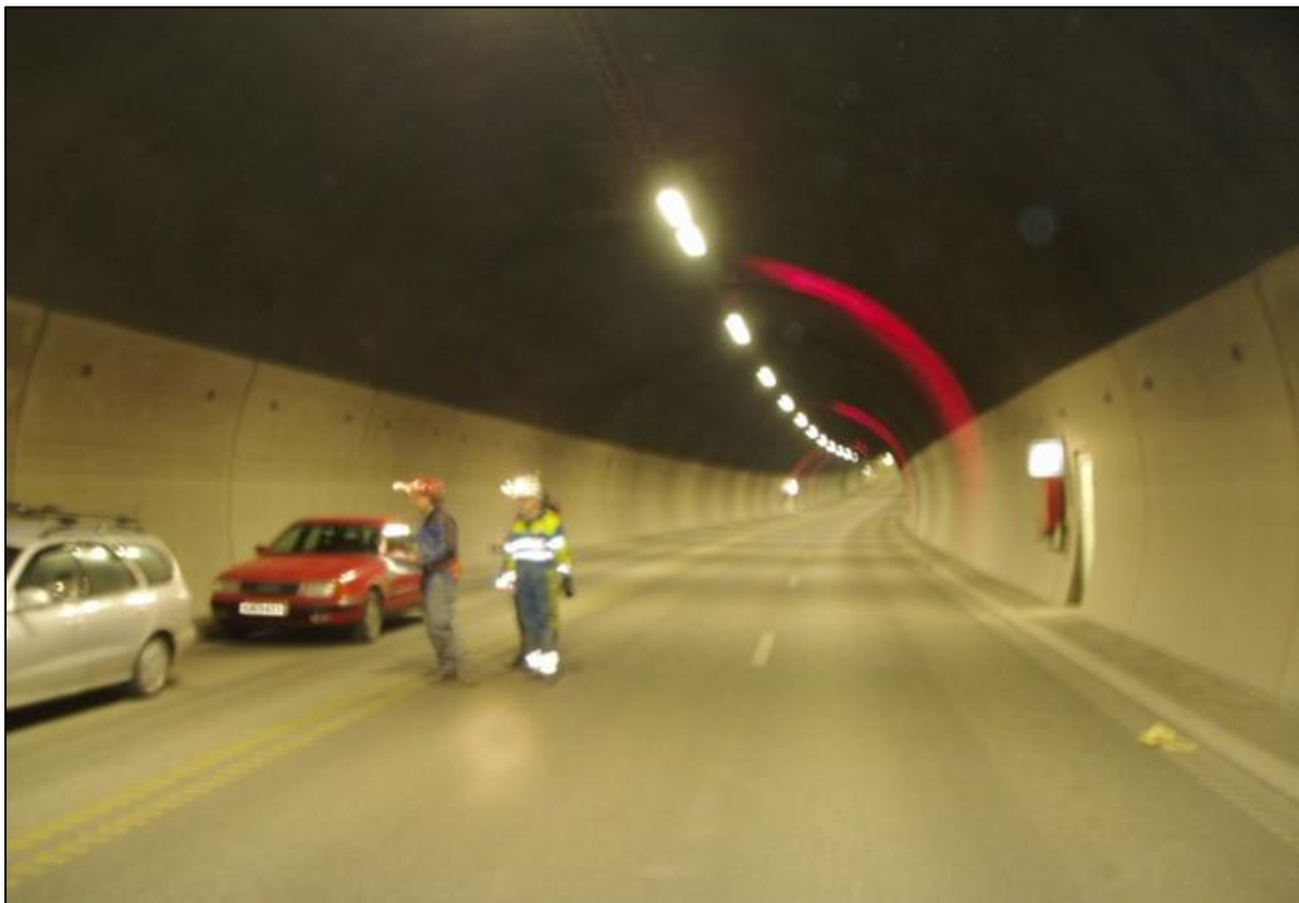
Common concept for rock support and water/frost lining of Norwegian road tunnels: drained tunnel, minor controlled inflow behind lining is accepted-
