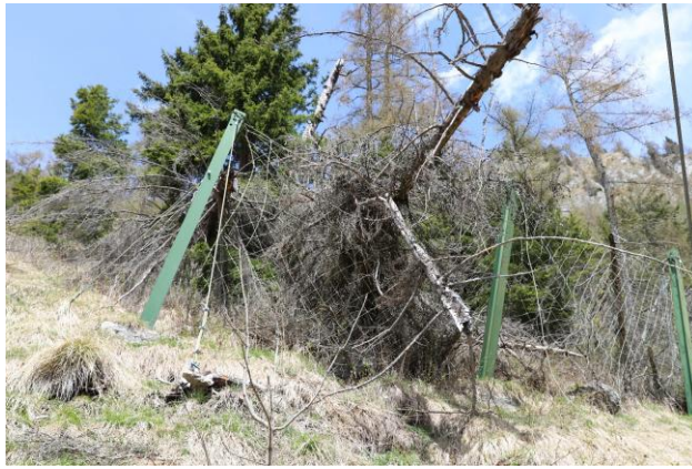
Fig. 2 Photograph of the first surveyed barrier: it appears highly damaged. In some sections, it has been completely torn apart. On the right is the classification in terms of LoC, %D and MCE.
