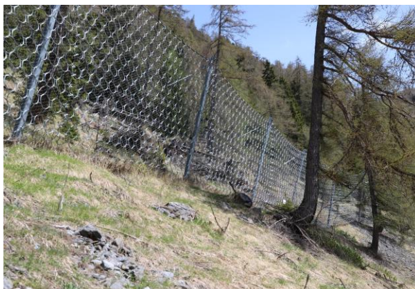
Fig. 3 Photograph of the second surveyed barrier: it appears in very good conditions, although pine trees grow very close to the structure. On the right is the classification in terms of LoC, %D and MCE.
