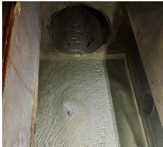
Fig.: Sinter formations in a drainage shaft inside the Gotthard Base Tunnel and heavily sintered pipe (Source: Harer)
