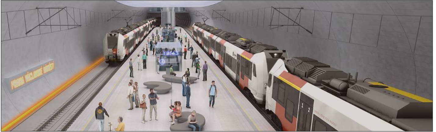
Figure 8: Visualization of single-aisle mined station with suburban regional trains. Source: Správa železnic, státní organizace.
