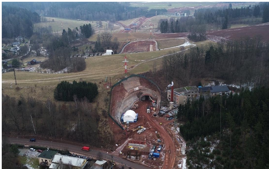
Figure 3: View of the Dolní Radechová Tunnel alignment (foreground: Dolní Radechová portal)
