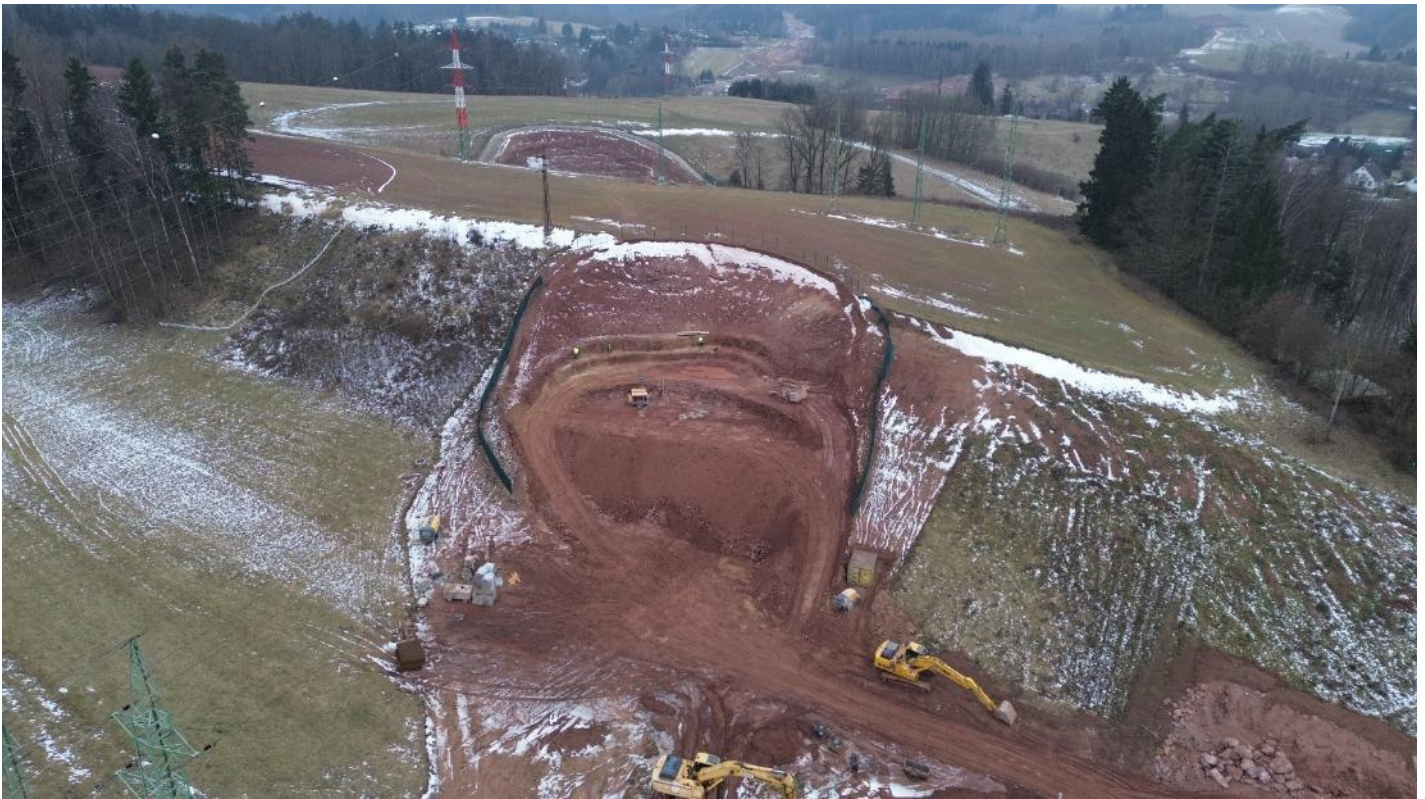
Figure 12: View of the Babí portal
