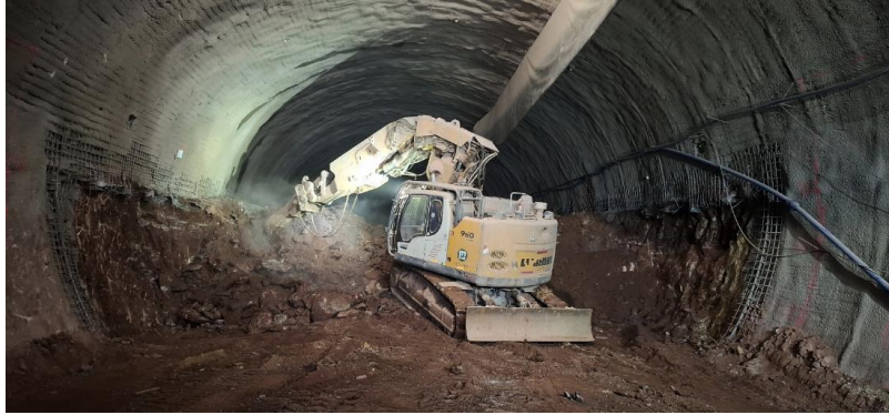
Figure 4: Bench excavation in Section 1
