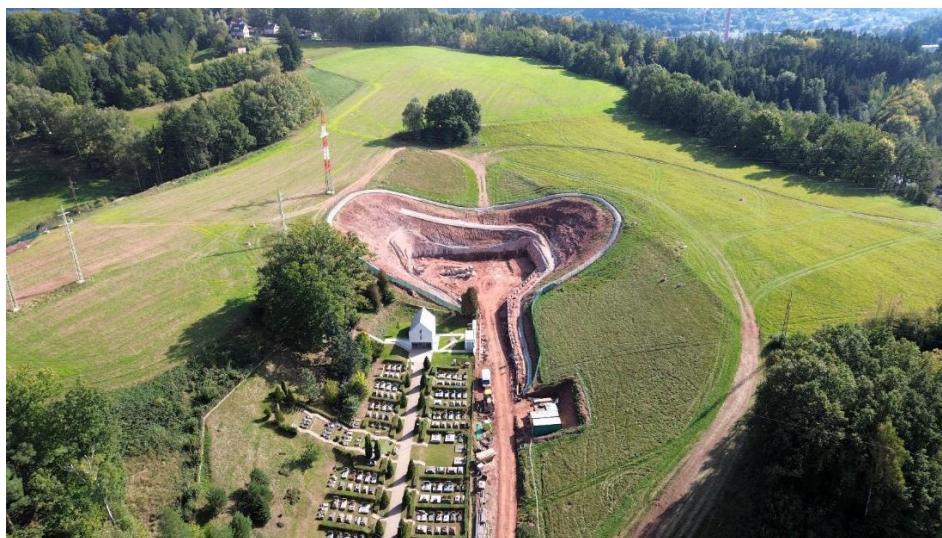
Figure 9: View of the excavation pit – middle section
