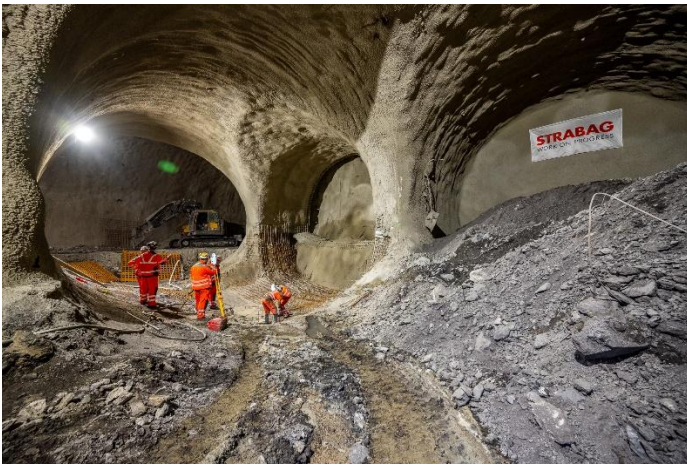
Figure 5: Surveying of truss frames at the bottom of the south station connecting tunnel
