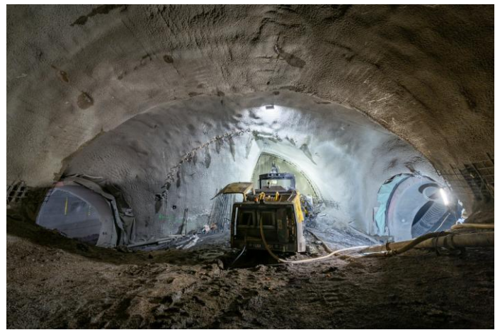
Figure 6: Drilling of face anchors in the production tunnel
