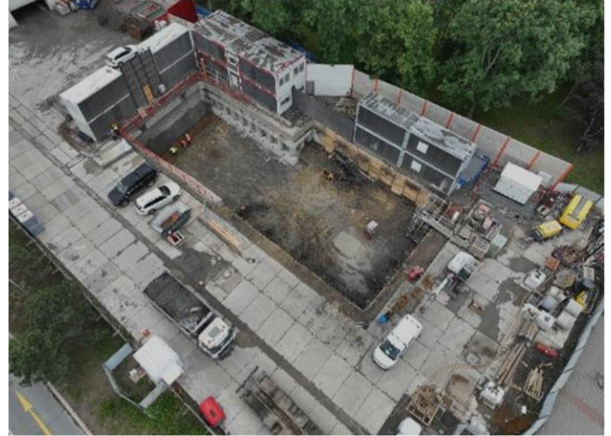
Figure 10: A drone view into the pit of the north vestibule, showing sound-absorbing cladding on the noise barriers during the grouting of the micro-pile umbrella for the north escalator tunnel
