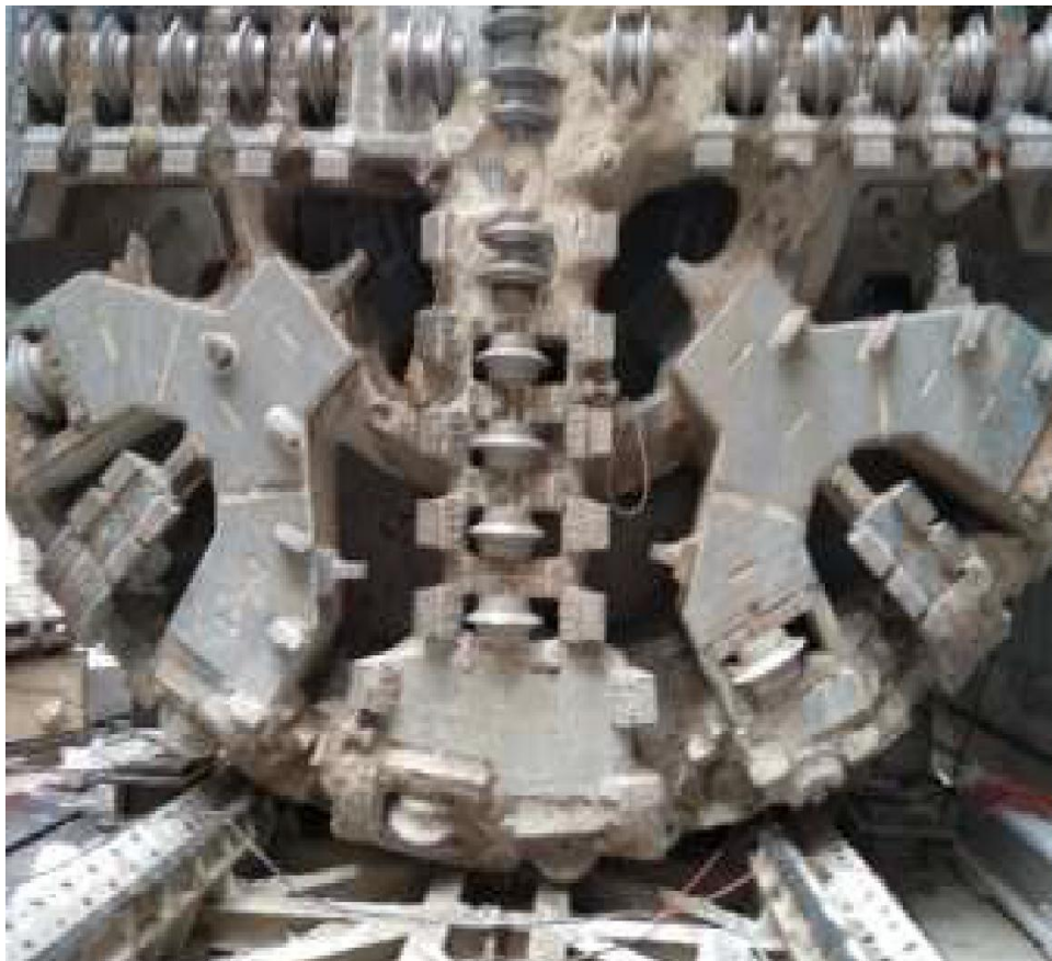
Figure 6. Picture taken during a site inspection before a relaunching.
