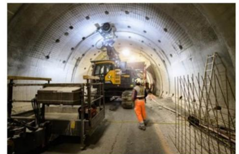
Figure 5: Controlled milling of the non-reinforced concrete tunnel lining
