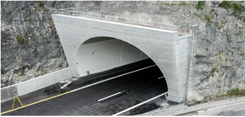
Figure 31: Finished portal of tunnel T3 (©patriceschreyer.com)
