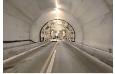
Figure 30: Traffic circulation with formwork in place during renovation works
