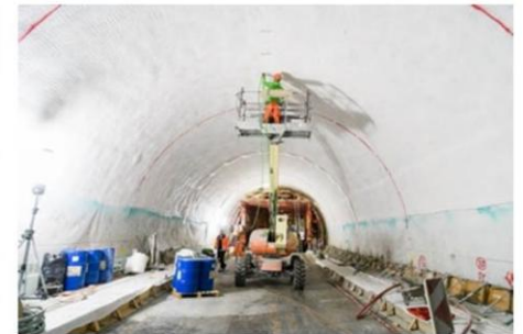
Figure-8:-Spray-on-waterproofing-system· (©patriceschreyer.com)
