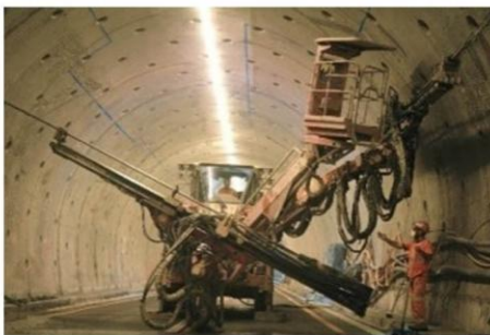
Figure 25: Drilling works inside the tunnel during night-time closures
