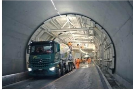
Figure 29: Inner lining casting with mobile curing and formwork units
