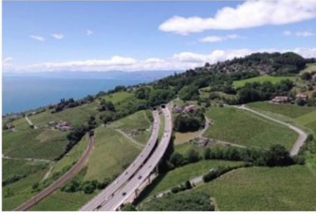
Figure 22: Project area of the Criblette and Chauderon tunnels
