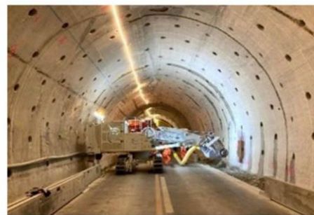
Figure 26: Controlled removal of the existing lining
