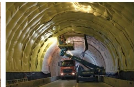
Figure 27: Installation of waterproofing system
