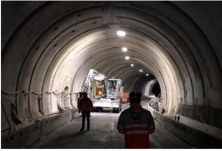
Figure 13: Night-time works inside the tunnel during renovation
