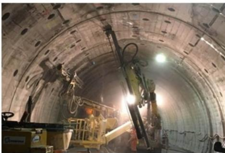
Figure 4: Installation of temporary rock bolts to stabilise the tunnel arch after milling
