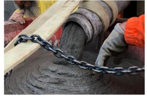
Figure 15: Fresh UHPFRC consistency during casting
