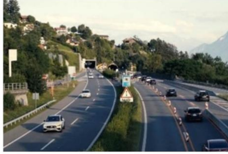
Figure 23: Traffic management layout on the A9 motorway during renovation works
