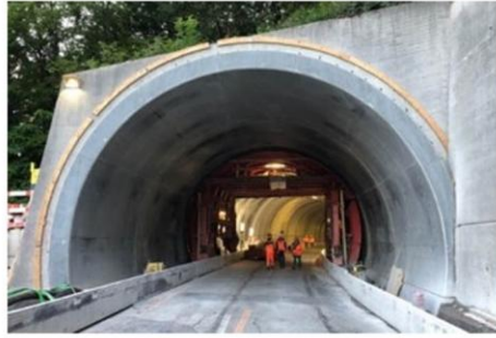
Figure 14: Completed inner lining after renovation
