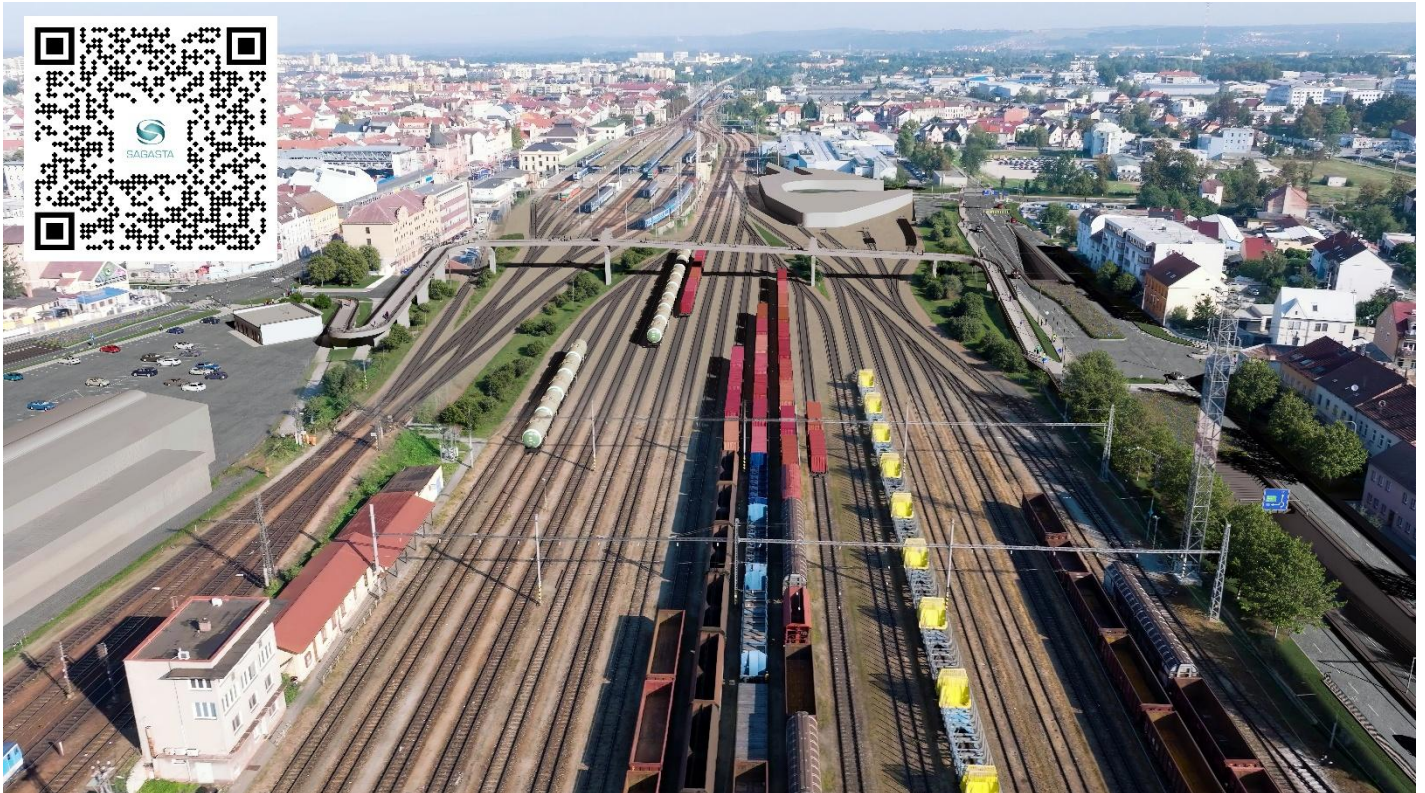
Figure 6: Overall view of the completed construction from the south
