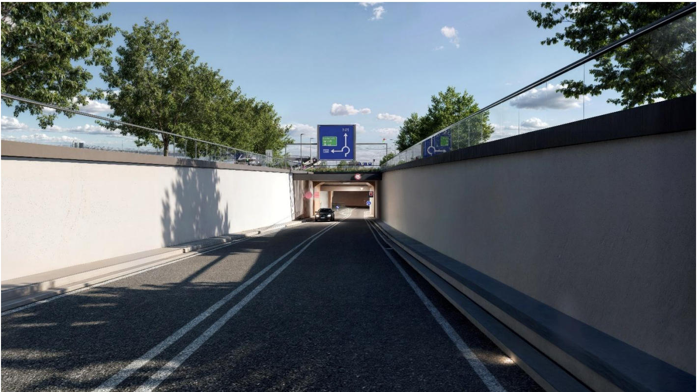
Figure 4: View from the U Lávky ramp to the "East" underground intersection
