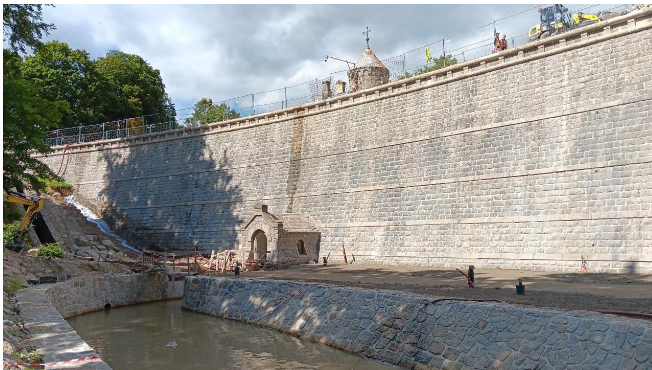
Fig. 10 Air side of the dam
