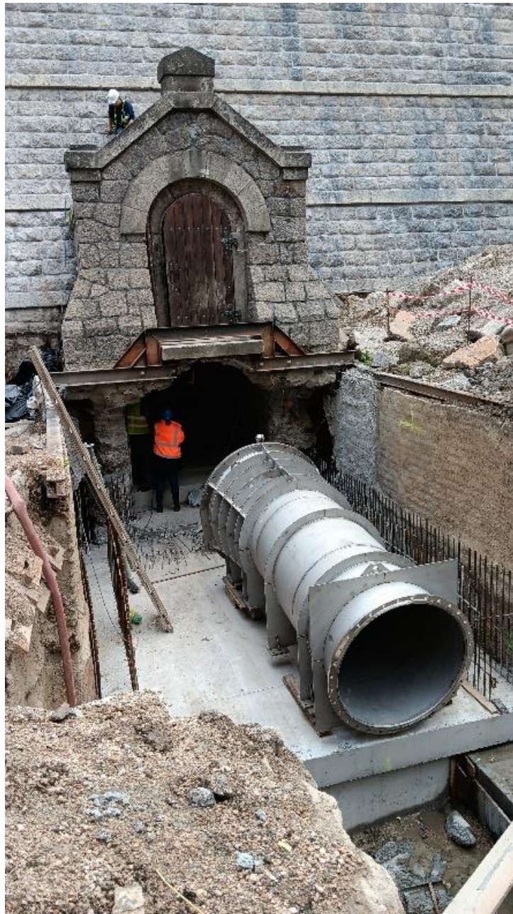
Fig. 9 Installing the bottom drain segment DN1200
