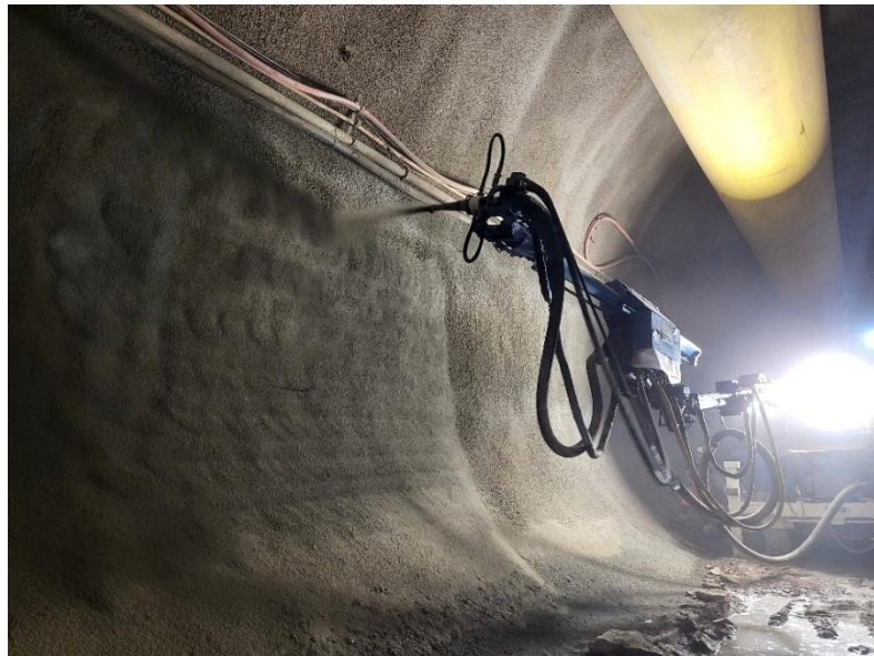
Figure 7: Spraying a consecutive block adjacent to the one in the first third of the picture without visible seam at the transition
