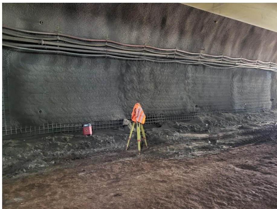
Figure 6: Consecutive areas (blocks) of the sidewall; seams at transitions and herringbone pattern visible
