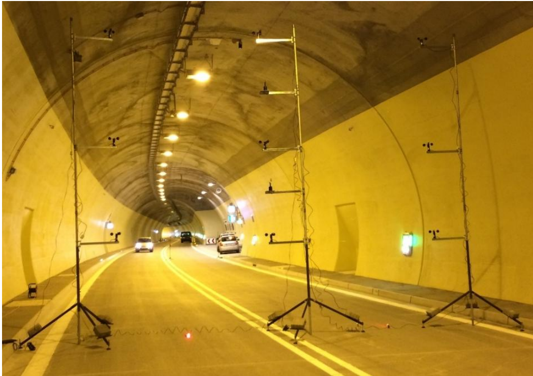
Figure 4: Network measurement of airflow in Poľana tunnel
