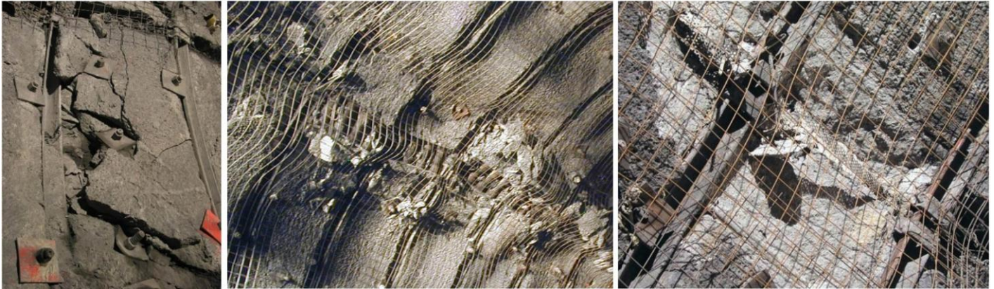
Figure 15: Behaviour of convergence slots – sliding joints (left), spring pots (centre), crushable concrete blocks (right)
