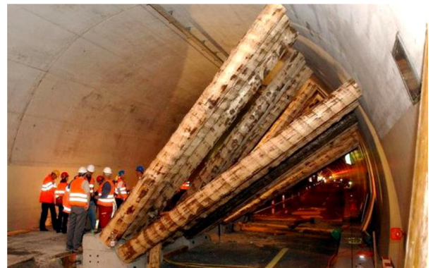
Figure 4: Temporary propping of the gallery to stabilize the flexural shear crack
