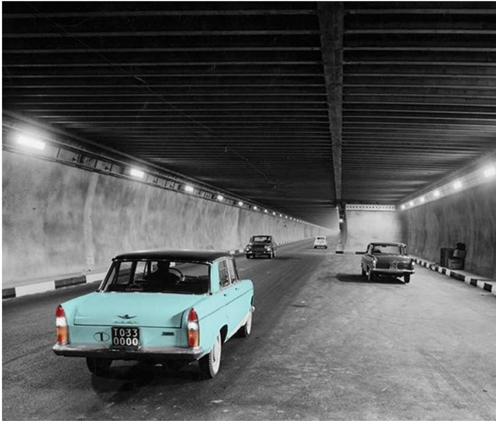
Figure 1: Gei Tunnel Switzerland opened in 1967
