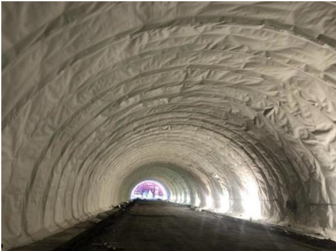
Figure 2: Fully bonded membrane ready for concrete application
