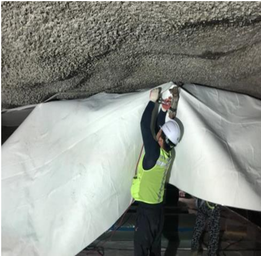
Figure 14: Fixation of the membrane using the geotextile
