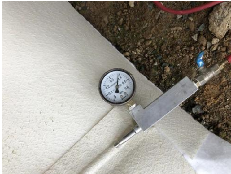
Figure 16: Test of welding seams
