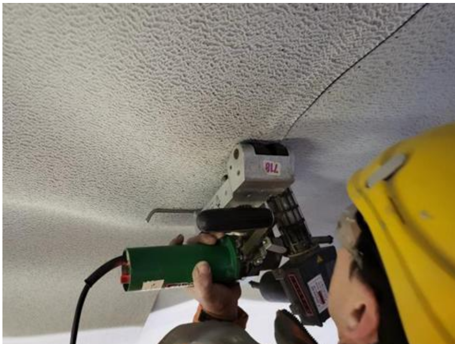
Figure 15: Hot air welding of the membrane
