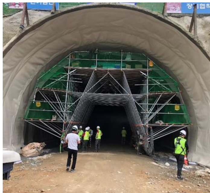
Figure 7: Tunnel in South Korea with SikaProof®-110
