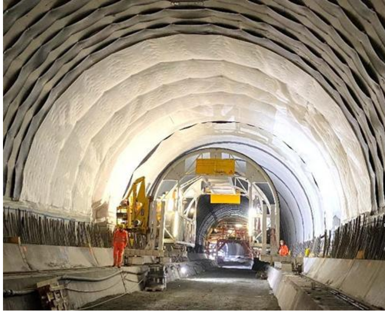
Figure 12: Scaffolding for membrane installation
