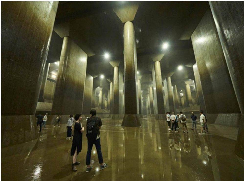
Fig 8 Tokyo's Metropolitan Outer Area Underground Discharge Channel – one of the world largest flood controls
