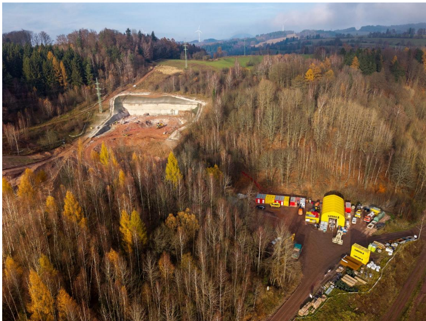
Figure 3: Construction site facilities near the southern portal of the Opevnění tunnel.
