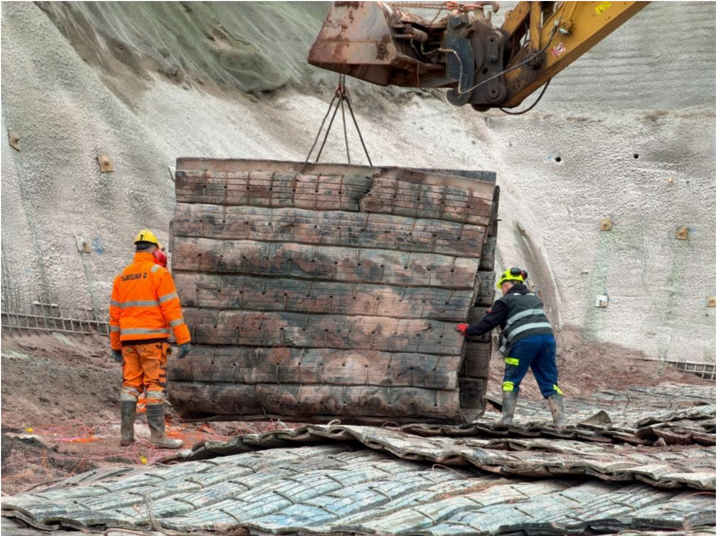
Figure 6: Use of protective mats as a measure during blasting works
